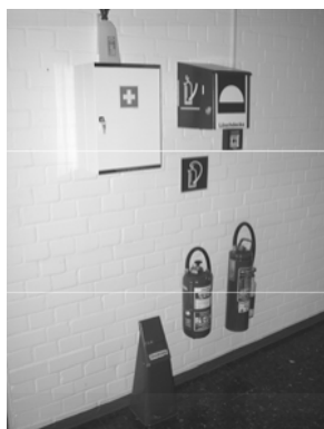
Fig. 1: Corridor in A
